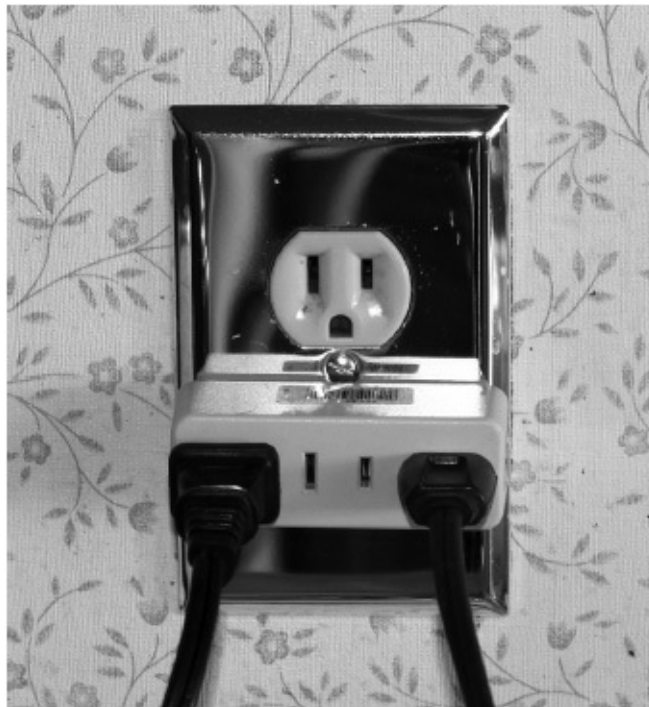
FIGURE 3-9 Proper use of a block tap in a 117-V electrical outlet.
