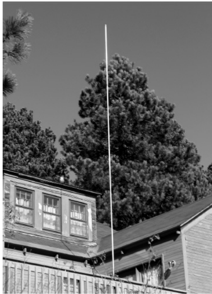
FIGURE 8-12 The antenna for the ham radio station shown in Fig. 8-11 . It's made of telescoping sections of aluminum tubing, mounted on a deck railing, and can be taken down or put up in a couple of minutes.
